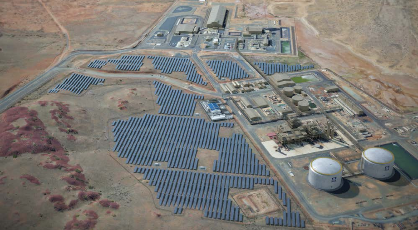
The Yuri renewable hydrogen facility in Karratha, Western Australia (site rendering). Image: ENGIE
